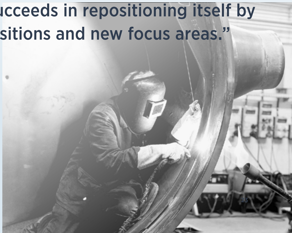
Welding work on a feedwater preheater for a nuclear power plant
